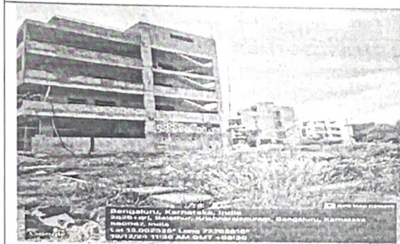
Residential houses are under construction
